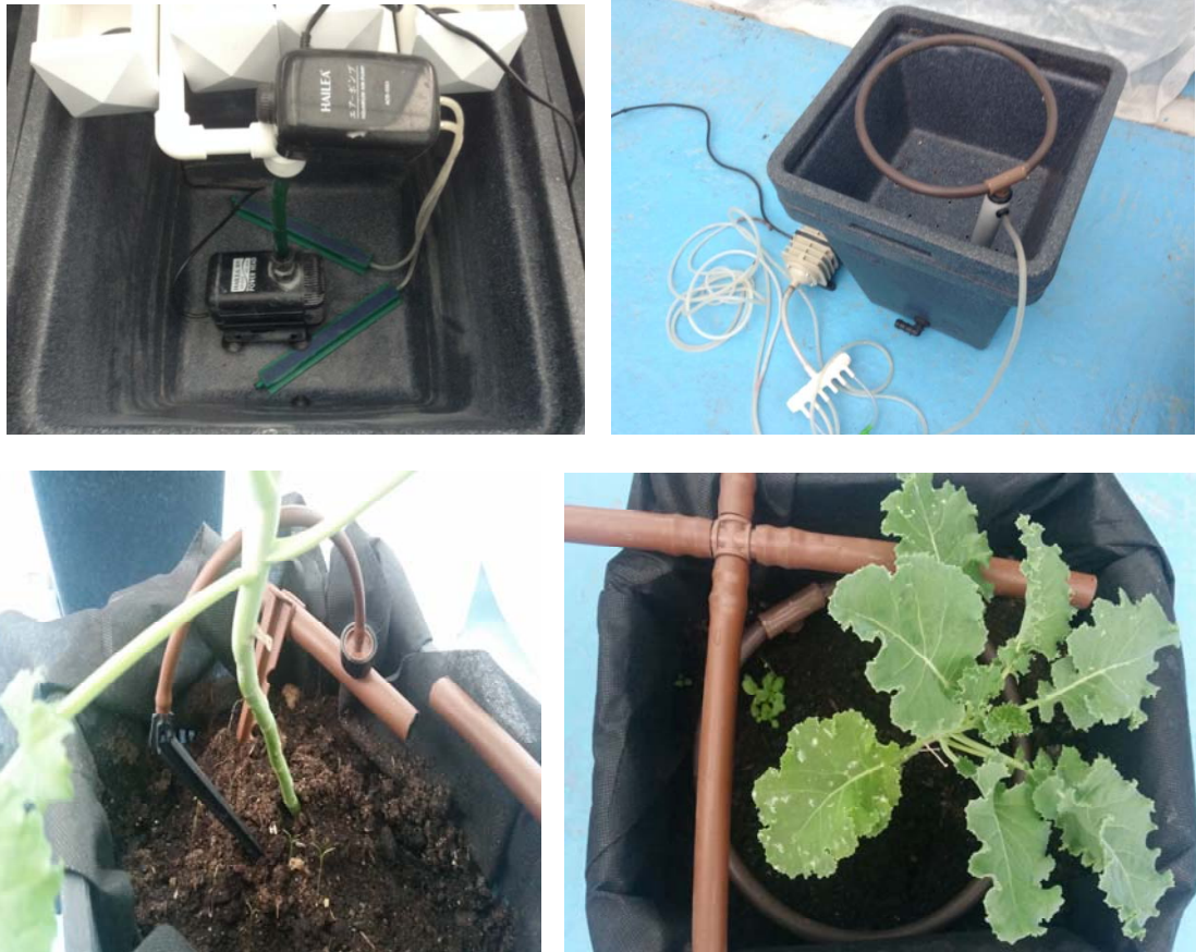
Photo 2 - Tank, water, and nutrient solution supply pump, as well as a drip irrigation system
